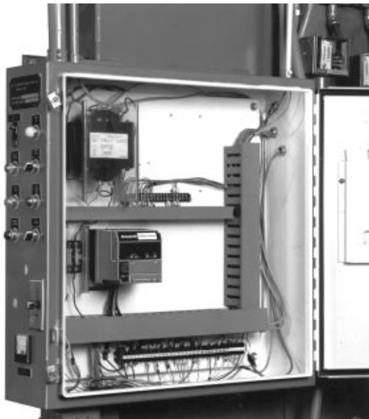
Fig. 7. Electrical panel installation.
